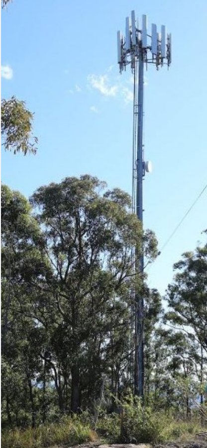
Securing mobile tower access
