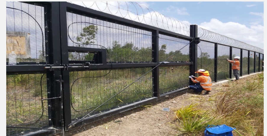
Security fence for rail corridor
